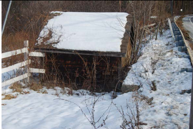
Photo 3. View looking east. Pump house. Main Street at right.
