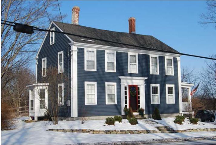
View looking north.
