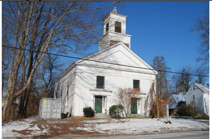
View looking north.
