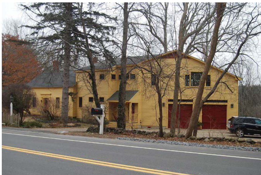
View looking southeast. Original main block at left.
