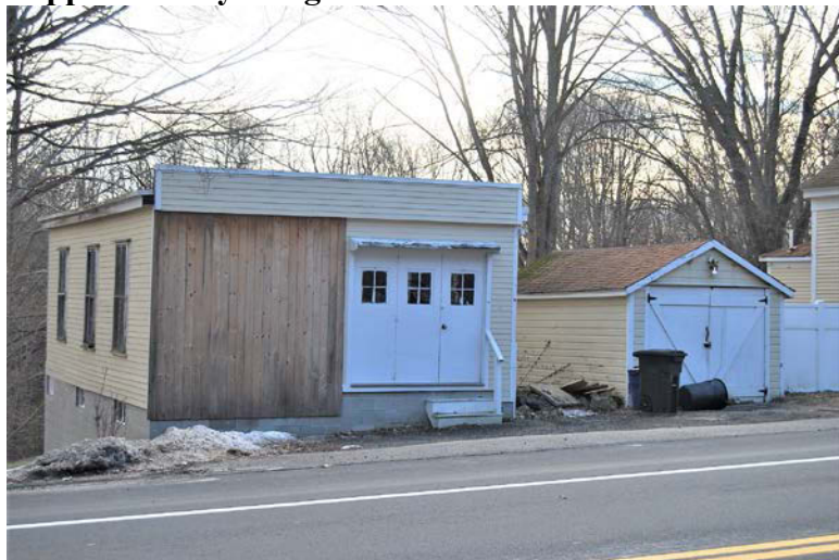
Storage building at left; garage (WNB.244) at right.
