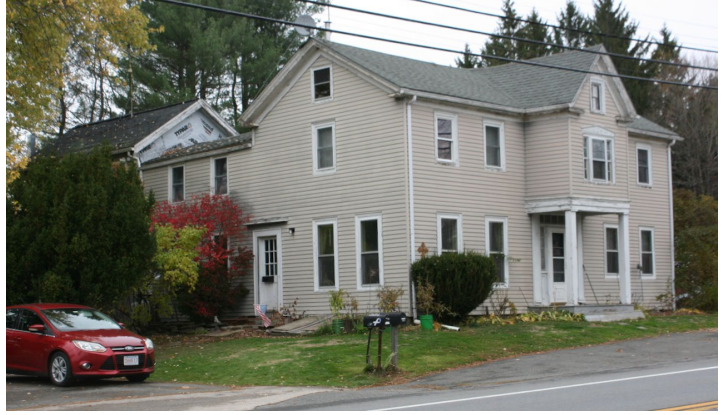
Photo 1. West and façade (south) elevations.
