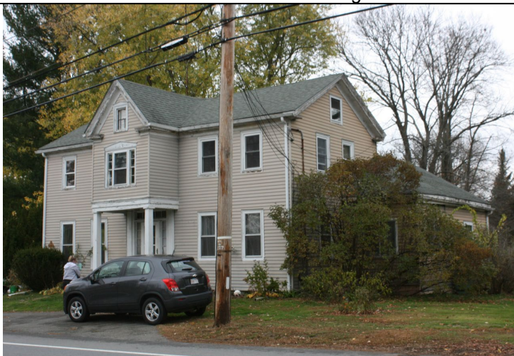
Photo 3. Façade (south) and east elevations.
