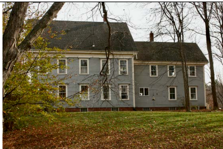
Rear (northwest) elevations of main block and ell.
