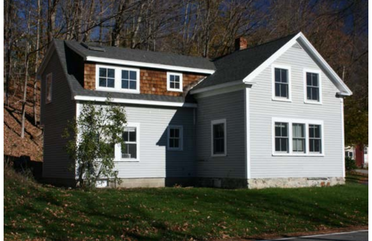
West and façade (south) elevations
