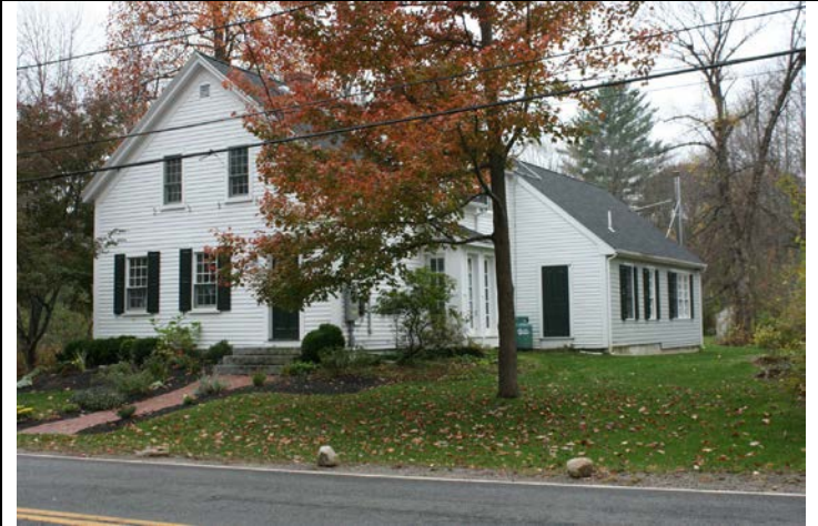
Façade (east) and north elevations.
