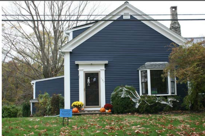
Façade (northeast elevation).
