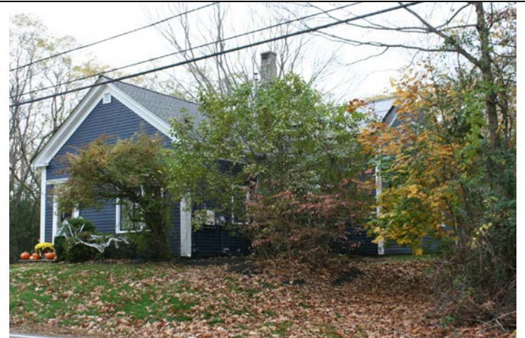
Façade (northeast) and right side (northwest) elevations.
