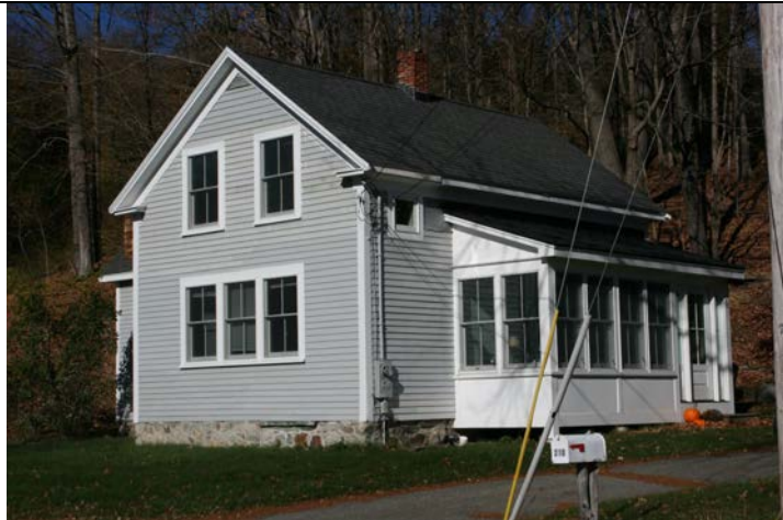
Façade (south) and east elevations of main block.
