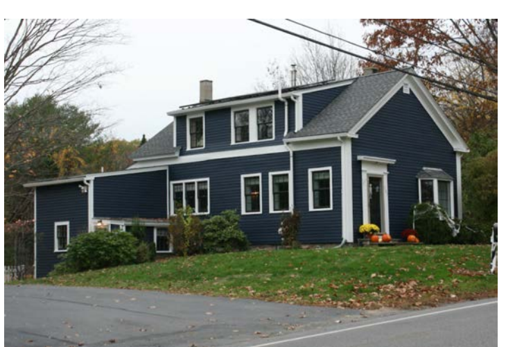
Right side (southeast) and façade (northeast) elevations.
