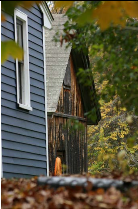
Barn: Northwest elevation.
