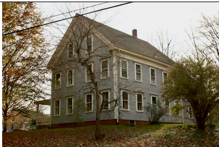
Side (northeast) and rear (northwest) elevations.
