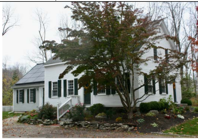
South and façade (east) elevations.
