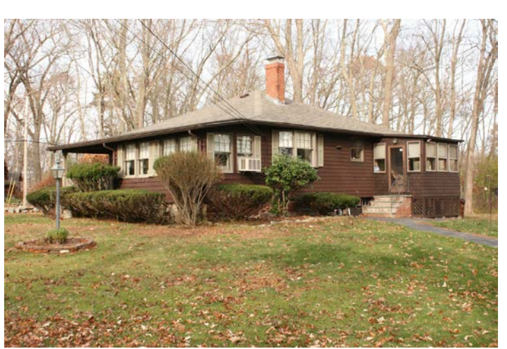
Façade (southwest) and southeast elevations.
