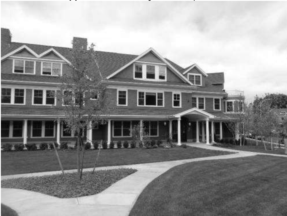
New construction in Brookline, MA 24 units on 1.1 acres Approximate density: 22 units per acre
