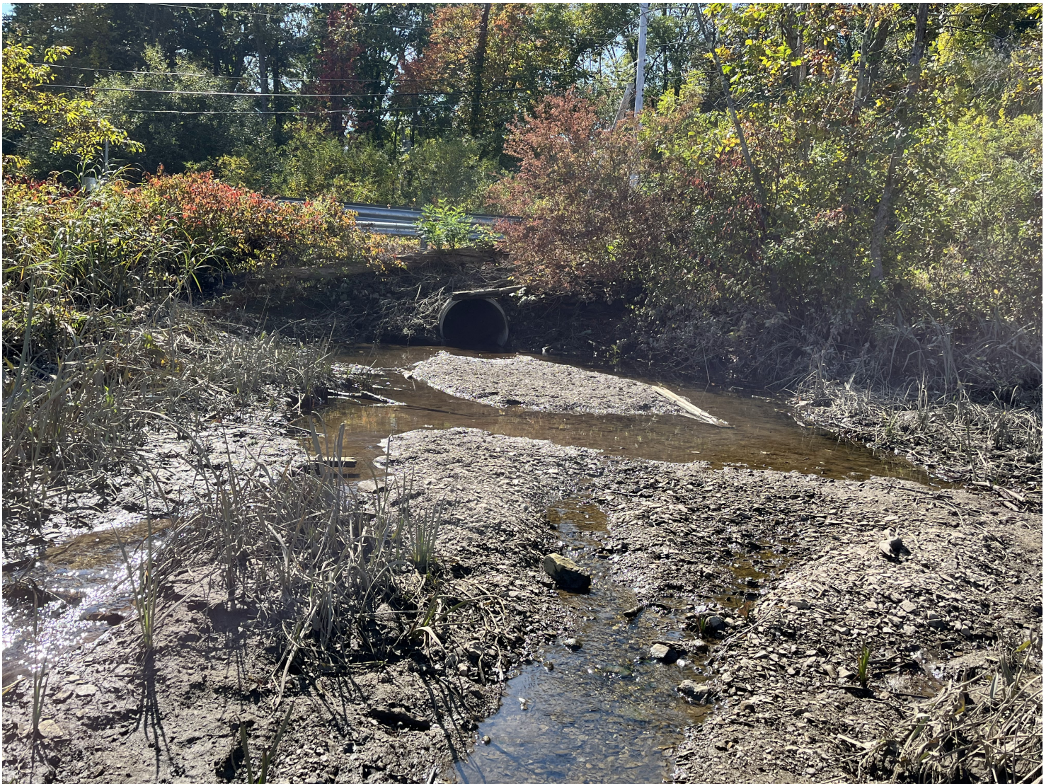
Outlet of culvert, note the proximity of utility lines and poles. 10/5/2023
