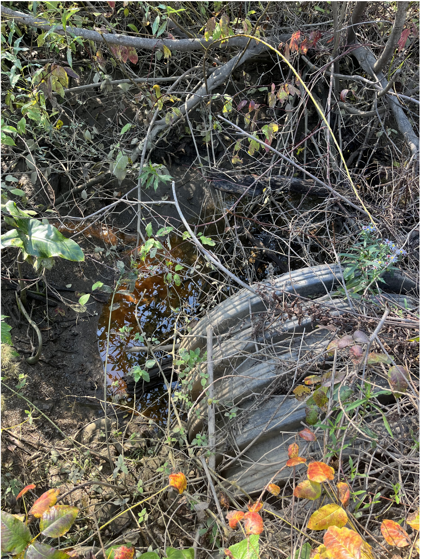
Inlet of culvert 10/5/2023
