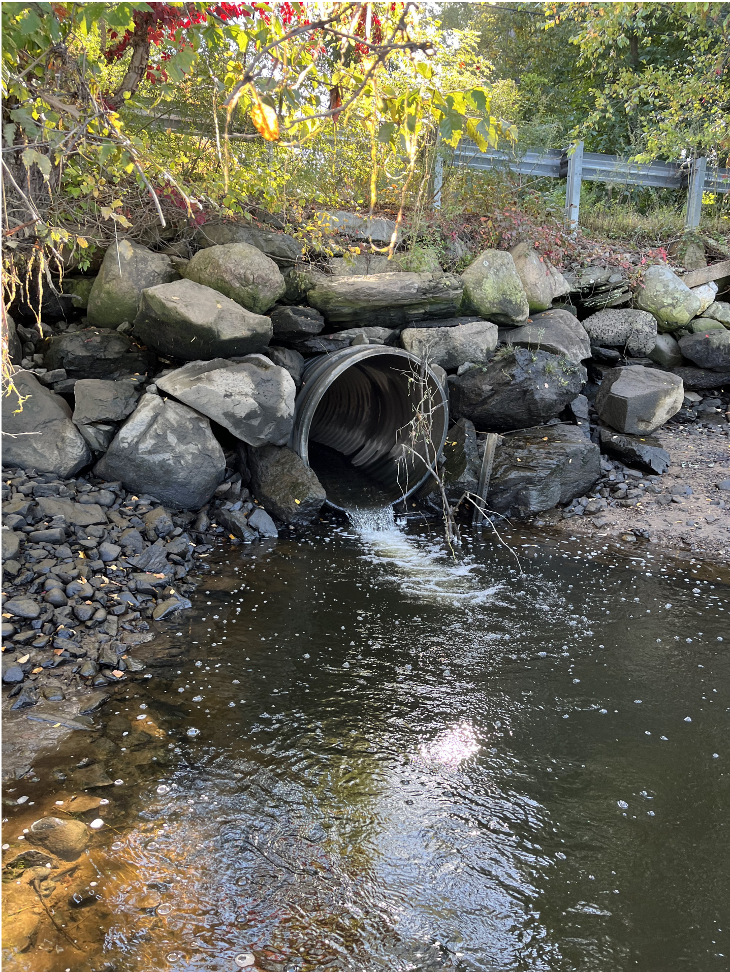
Culvert outlet at Merrimack River 10/5/2023
