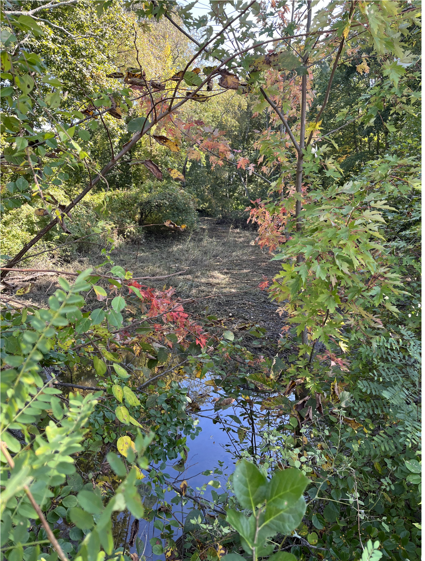
Inlet of culvert and tidally influenced perennial stream 10/5/2023
