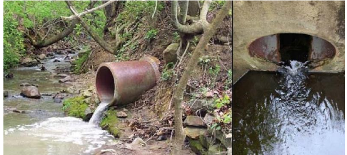
Combined sewer overflows in the Mystic River.
