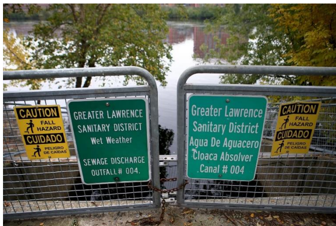
Combined sewer overflow outfall at the Greater Lawrence Sanitary District.
