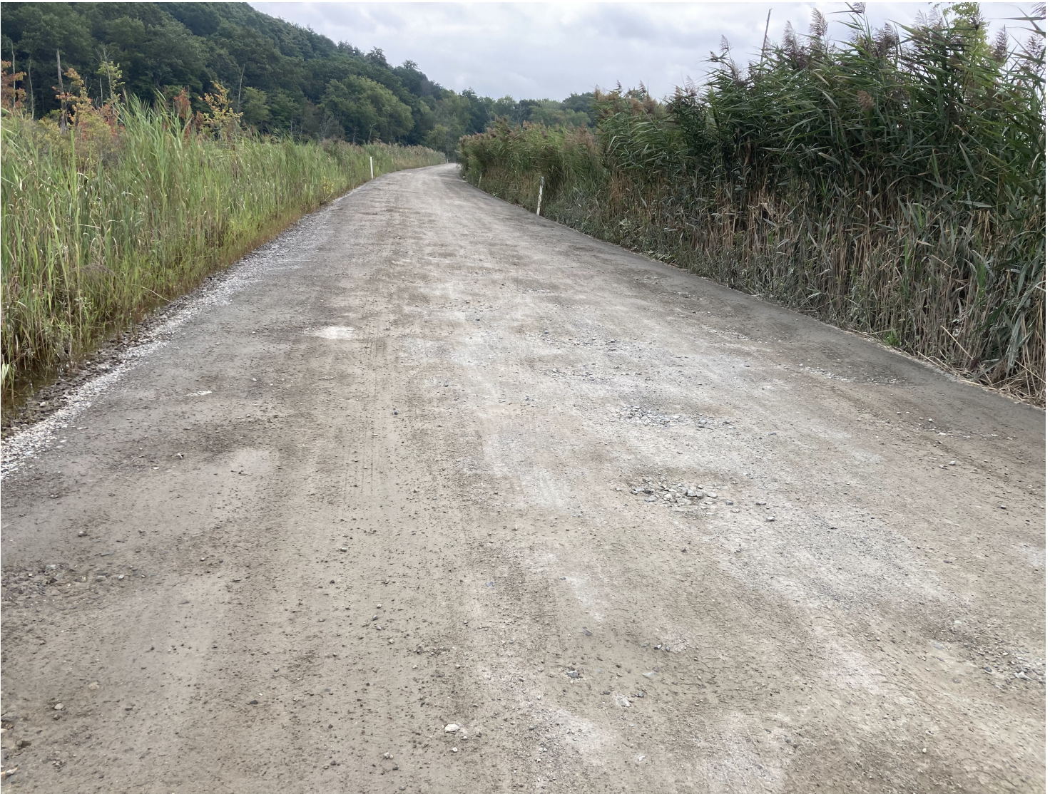
Existing Condition Photo 1: Gravel portion of Ash Street 9/8/2023
