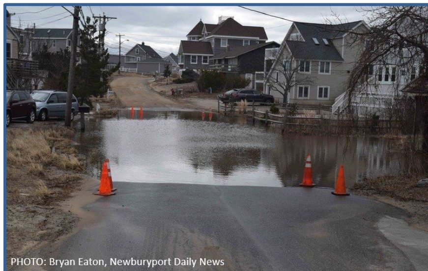
Figure 47. Water Table Ponding on Annapolis Way, March 5, 2018
