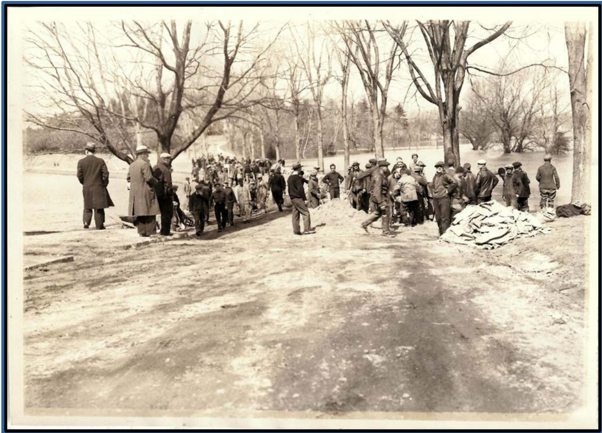
Figure 33. March 1936 Flood, volunteers build a berm to protect Bartlett Spring Pond
