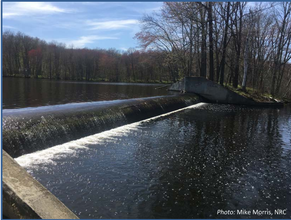
Figure 22. Lower Artichoke Spillway
