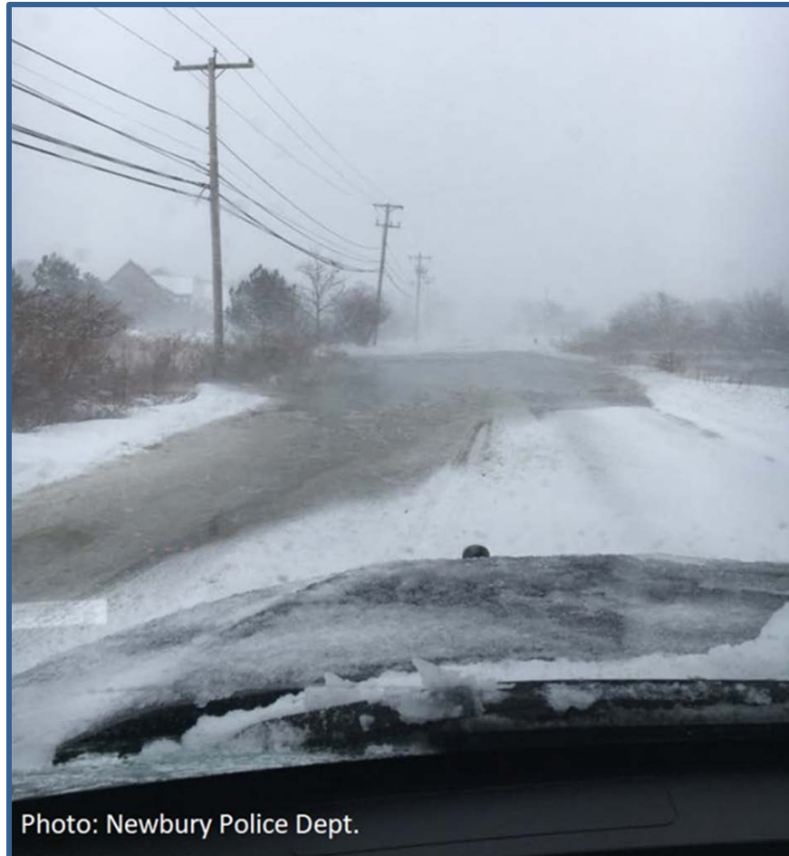
Figure 49. Plum Island Turnpike - Surge Flooding and Drifting Snow, January 4, 2018
