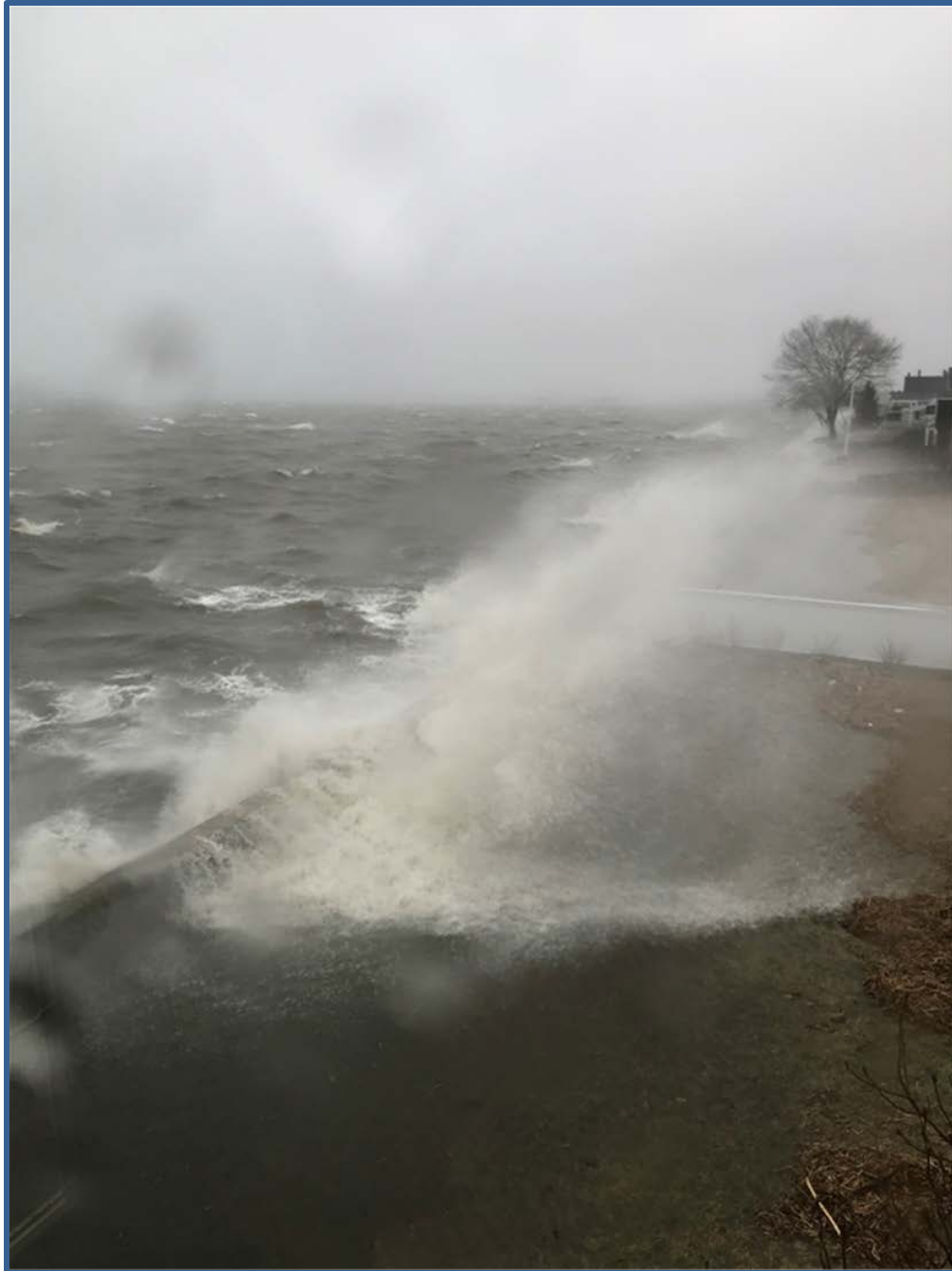
Figure 72. Wave Over-wash is Trapped behind Hale Park Seawall – Photo: John Morris
