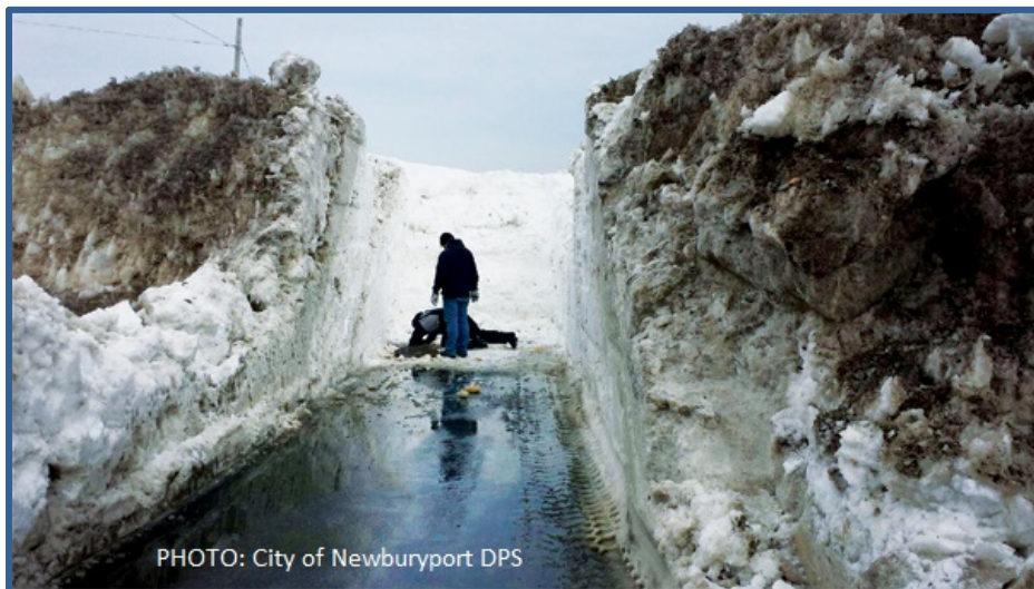
Figure 56. Winter Septic System Problems – Frozen Manholes
