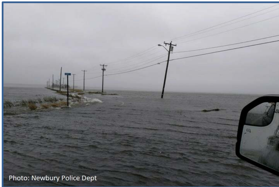
Figure 48. Plum Island Turnpike - Surge Flooding, March 3, 2018
