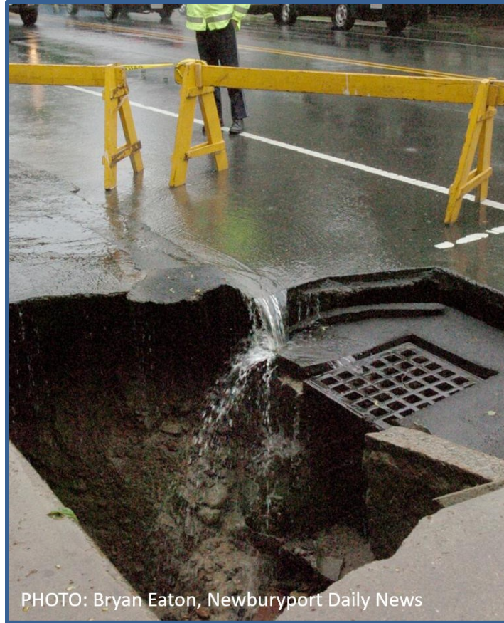
Figure 108. Storm Drain Sinkhole - Created by Heavy Rains
