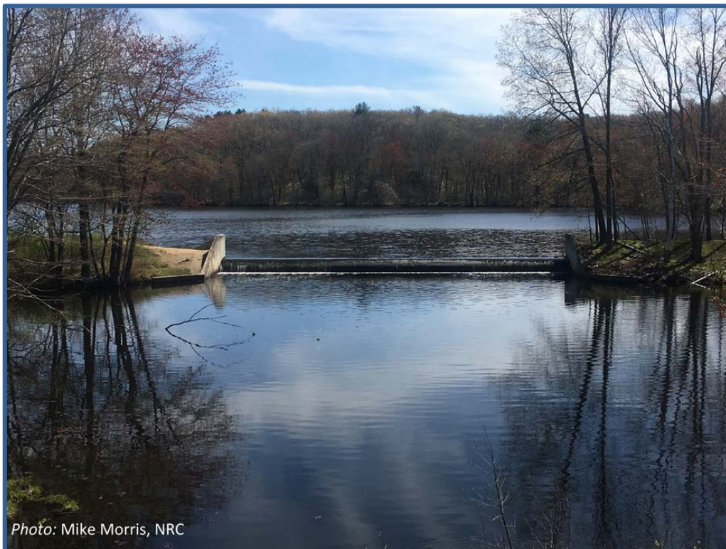
Figure 23. Lower Artichoke Spillway
