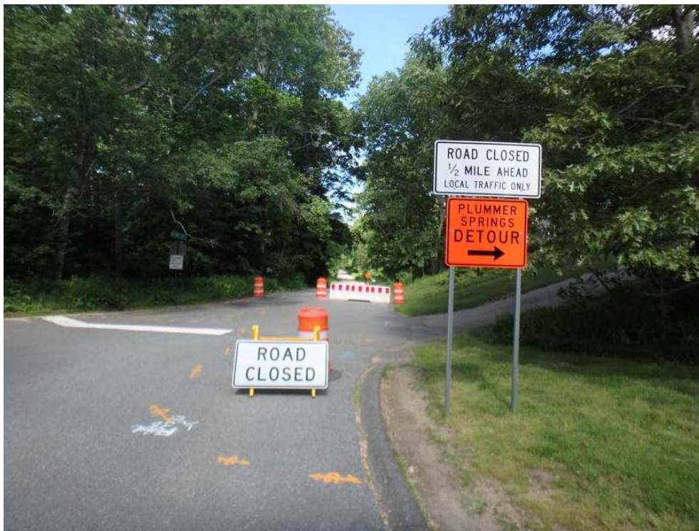
EAST ADVANCED BRIDGE CLOSURE SIGNAGE
