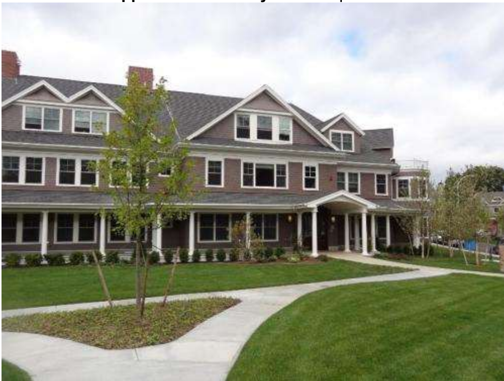
New construction in Brookline, MA 24 units on 1.1 acres Approximate density: 22 units per acre
