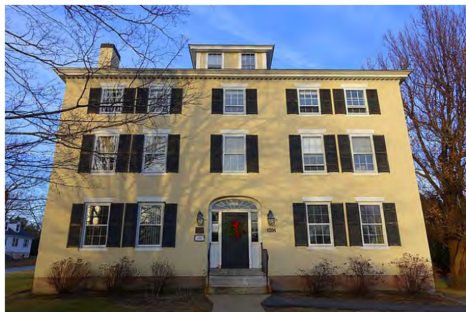
Starbard Administration Building.
