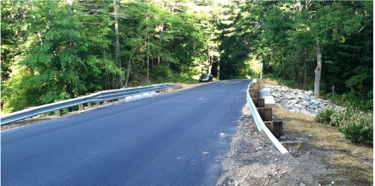
Thrie Beam – Guardrail Across Bridge
