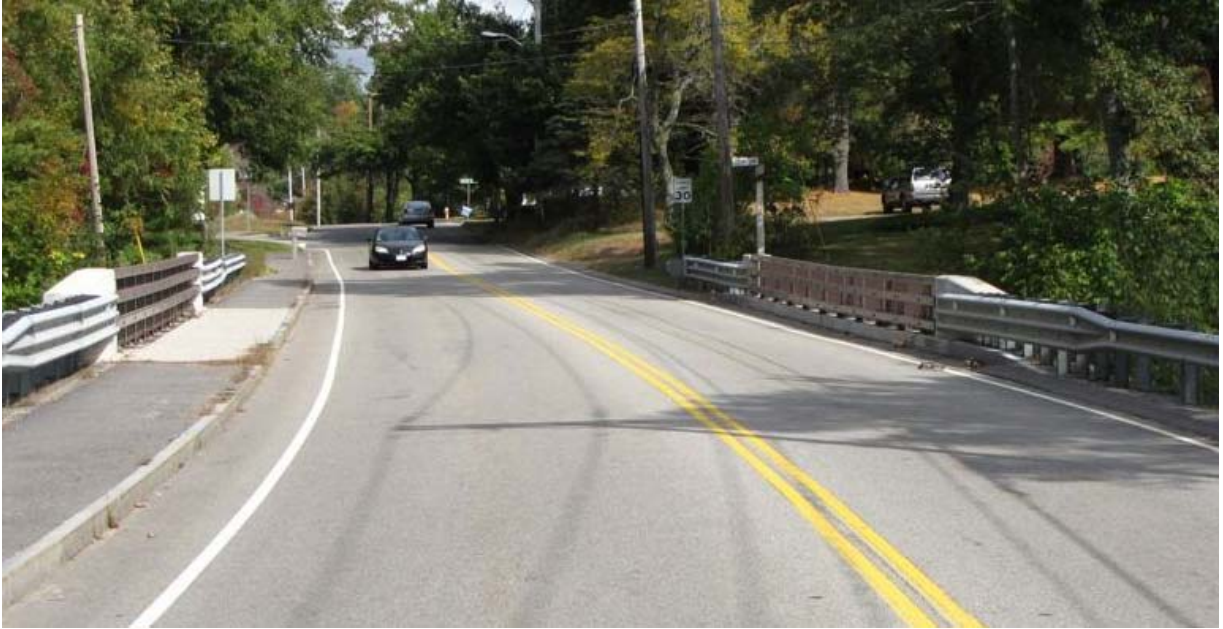
S3-TL4 – Bridge Rail & Concrete Transitions at Sidewalk
