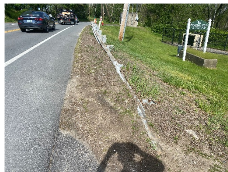
Image 5: Turned-down end treatment on approach side of Main Street.
