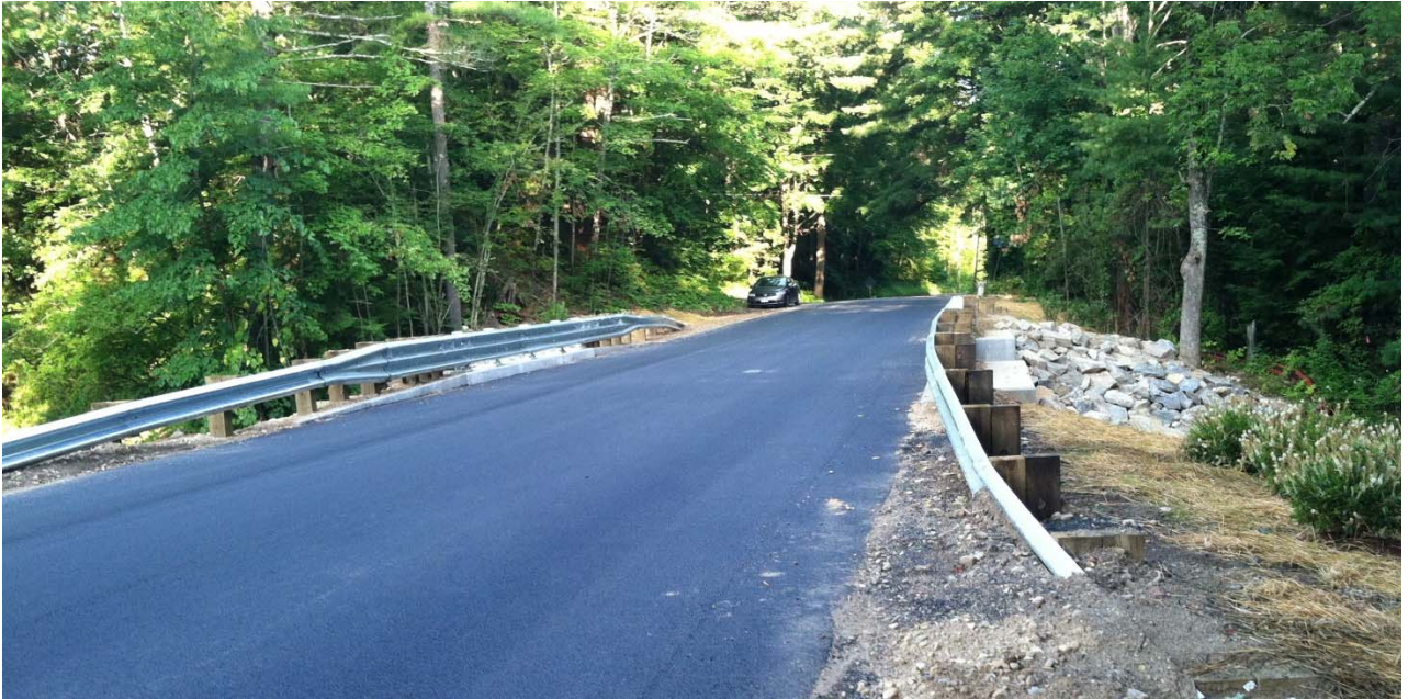
Thrie Beam – Guardrail Across Bridge
