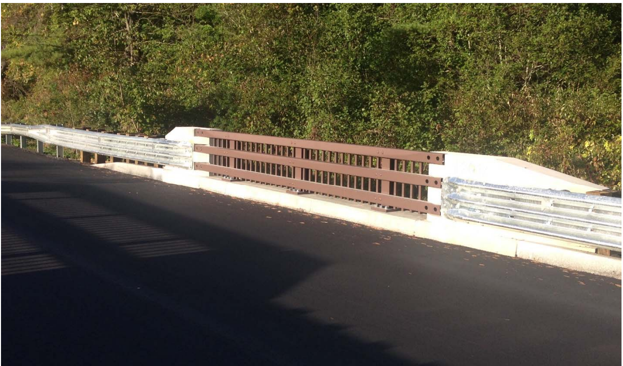
S3-TL4 – Bridge Rail & Concrete Transitions
