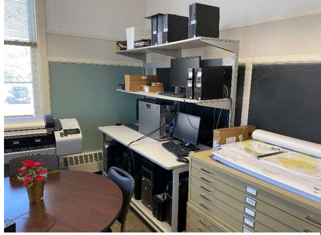
The existing network hub is located in a publicly-accessible location, presenting a security risk.
