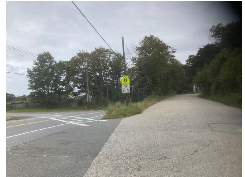
The access road has no sidewalk, yet a ladder-style crosswalk with reflective signage connects it to the recreational area located across Main Street. The crosswalk is at a right diagonal when exiting the access road.
