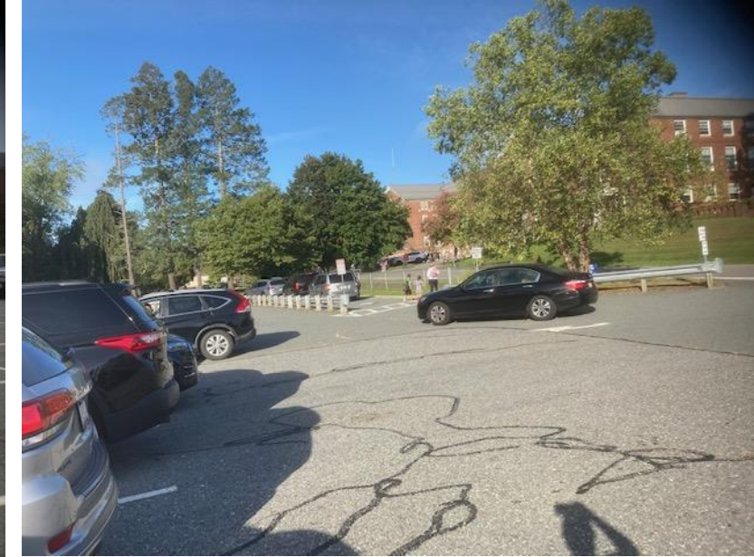
There is a conflict point near the school's arrival valet area. Here, parked family vehicles were observed leaving parking spaces unaware of oncoming vehicles. The expectation for parked vehicles is for vehicles entering the lot to use the valet area and not to park in the lot.
