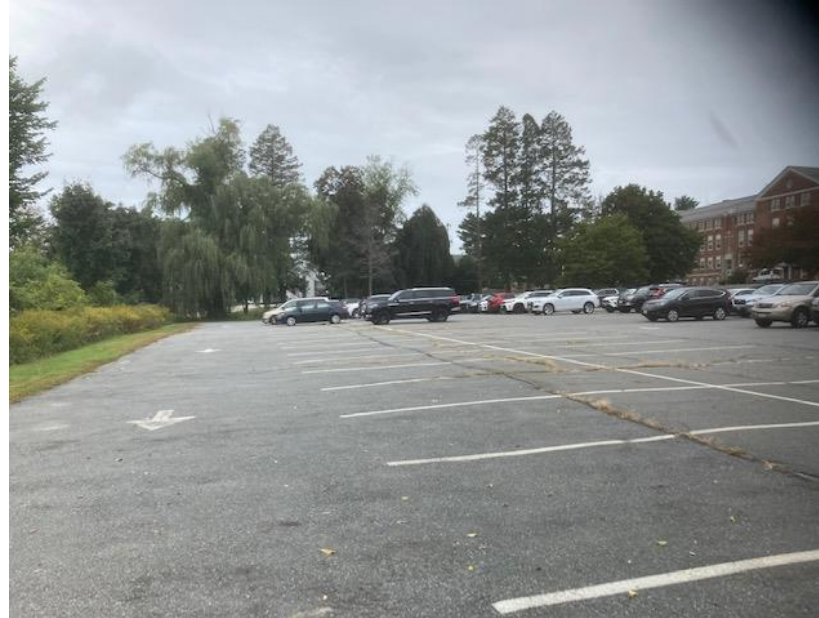
Directional pavement markings line the perimeter of the parking lot.
