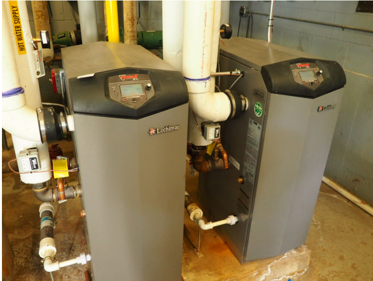
Figures 9a-b. Existing boilers assessed in site visit are relatively new, high efficiency units
