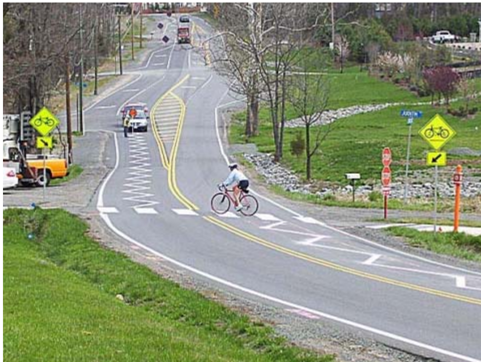
This photo shows another style of zig zag pavement marking tested in Virginia. Image from VDOT.
