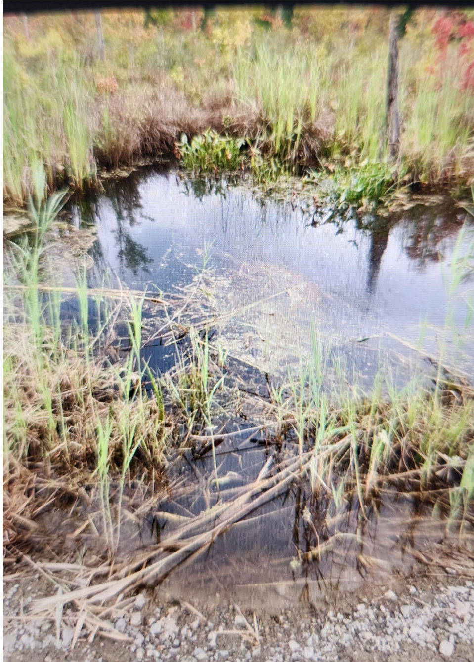
Existing Condition Photo 4: Area of culvert inlets
