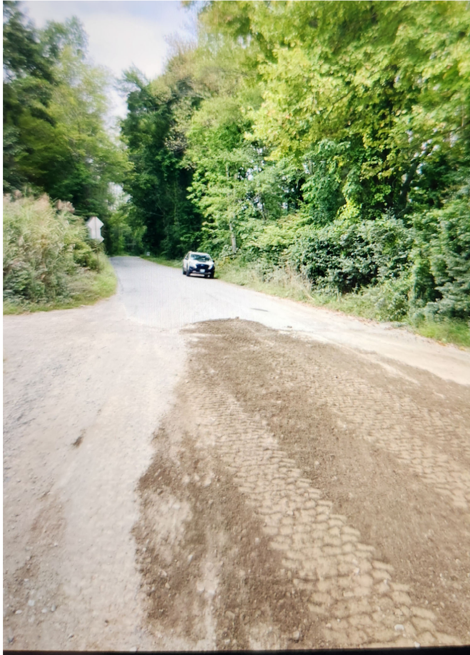
Existing Condition Photo 2: Gravel road meets paved road looking northwest. Area that appears "disturbed" is freshly spread gravel from 9/8/2023 emergency work.
