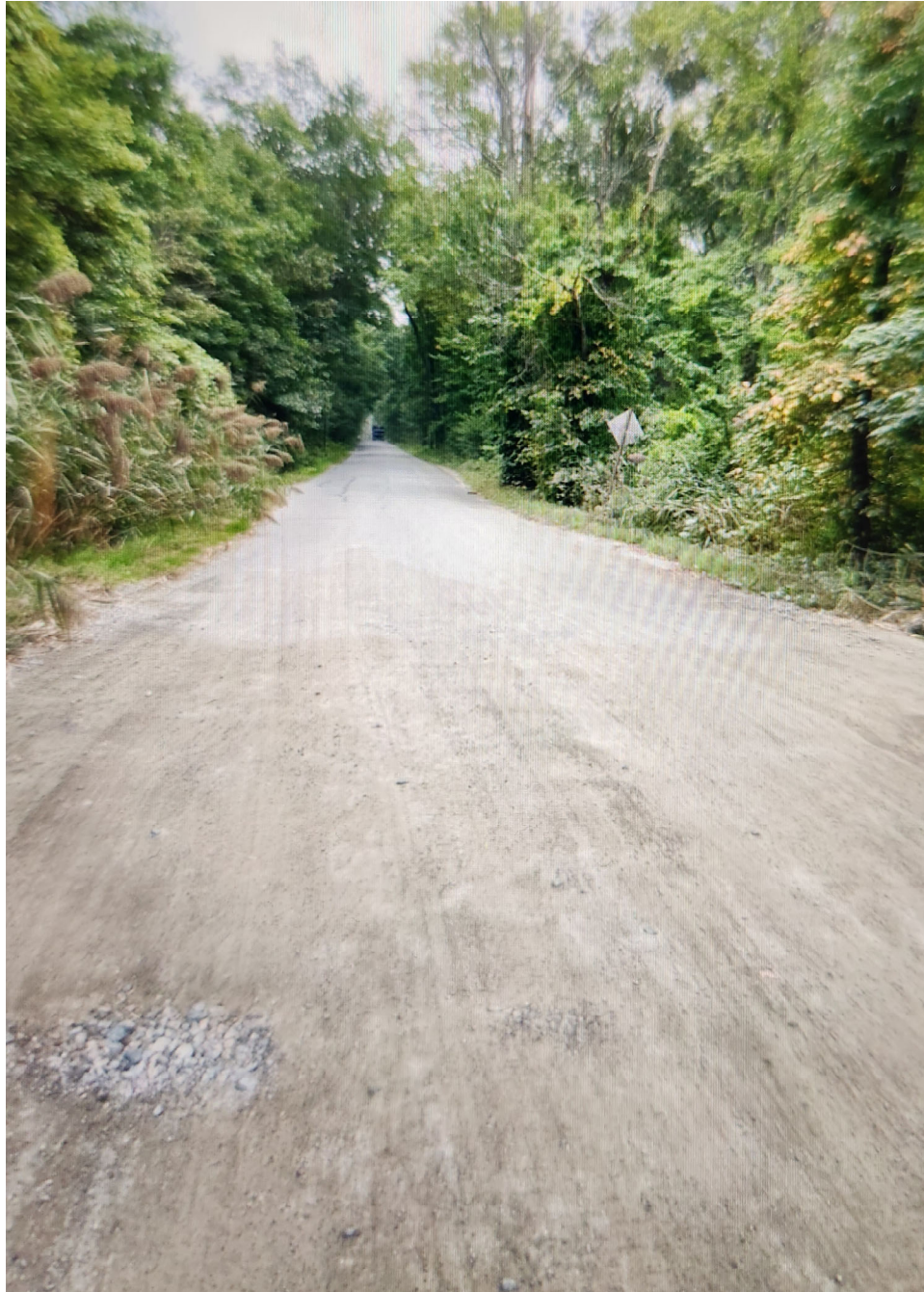
Existing Condition Photo 3: Gravel portion of road meets paved looking southeast
