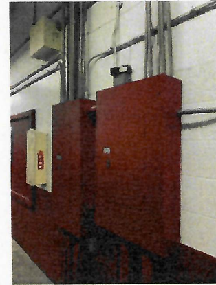
Non-ADA compliant electrical panels
