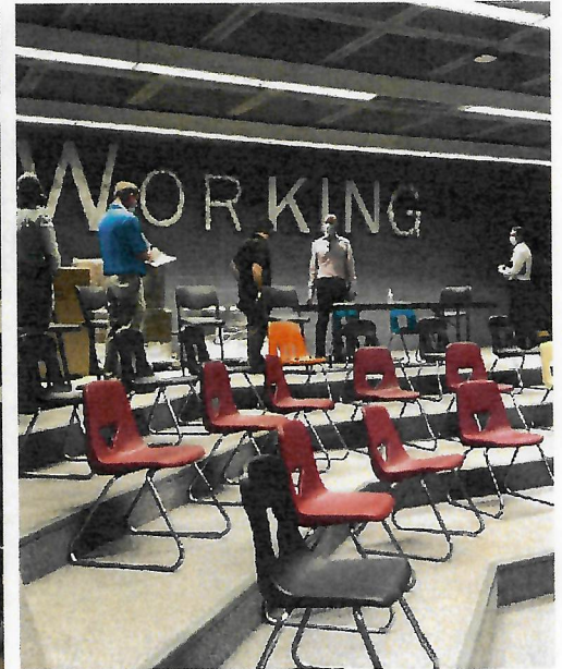
Tiered multi-purpose space without accessible route
