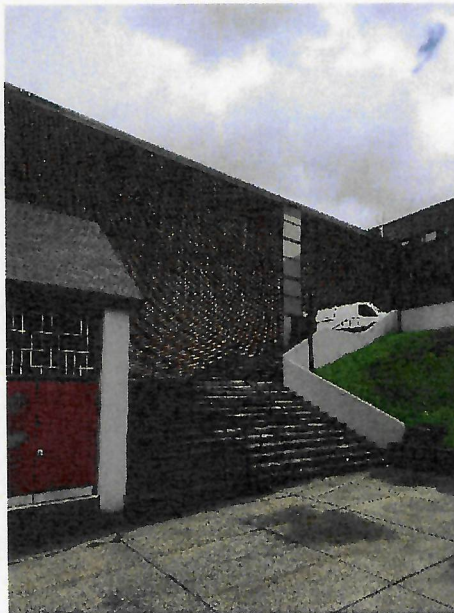
Lack of accessible route throughout the site
