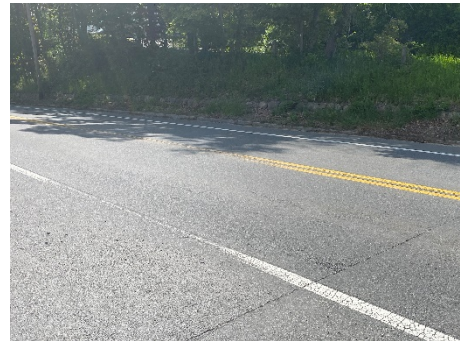
Image 3: Faded pavement markings along Main Street adjacent to Pipestave Recreation Area Driveway.
