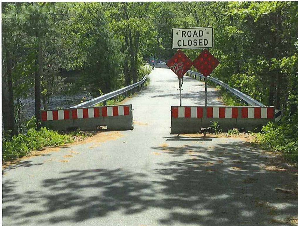
Photo 4: West approach Jersey barriers and "Road Closed" sign.
