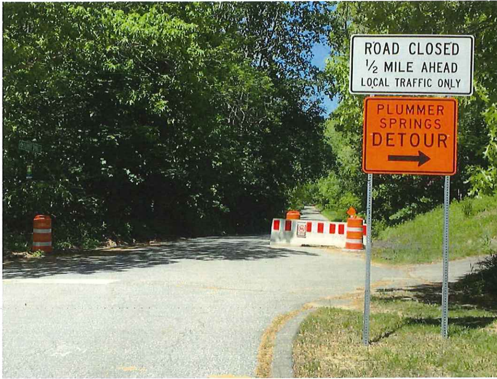
Photo 7: First advanced, "Road Closed" and "Detour" signs with Jersey barrier, east of the bridge.
