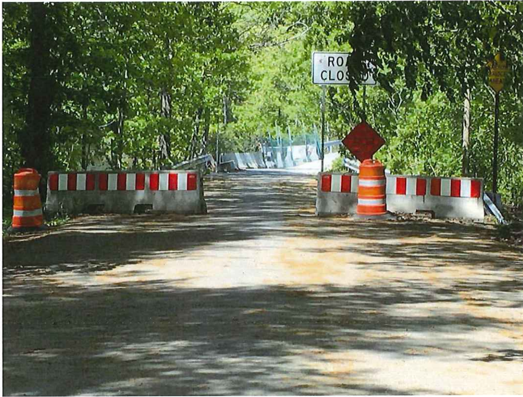
Photo 5: East approach "Road Closed" sign with Jersey barriers.
