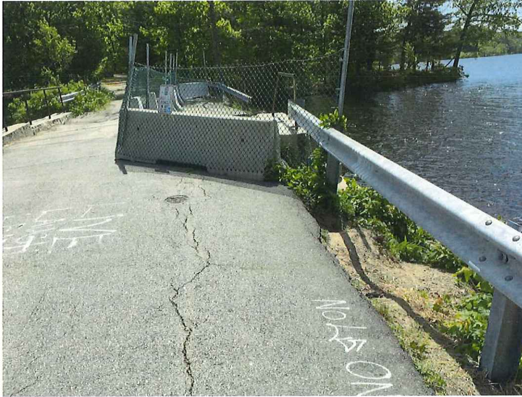
Photo 9: Jersey barriers with 6' high chain link fencing along the south side of the bridge. (West end shown, looking east).
