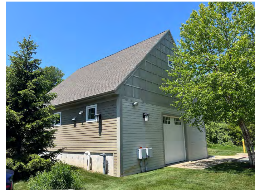
Wastewater treatment facility at Princeton Westford, a large multi-family development
