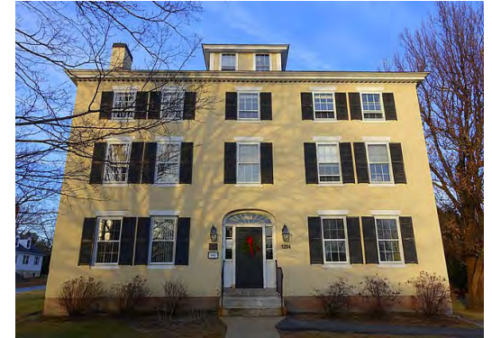
Starbard Administration Building.
