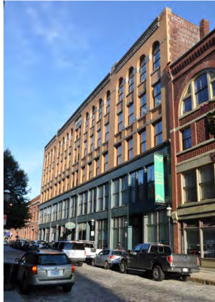
Pollard Exchange Building.
