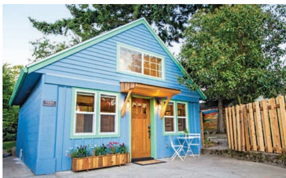
▲ Renting out this 350-square-foot garage-conversion ADU in Portland, Oregon, helps the property owner, who lives in the lot’s primary residence, pay her home mortgage.
