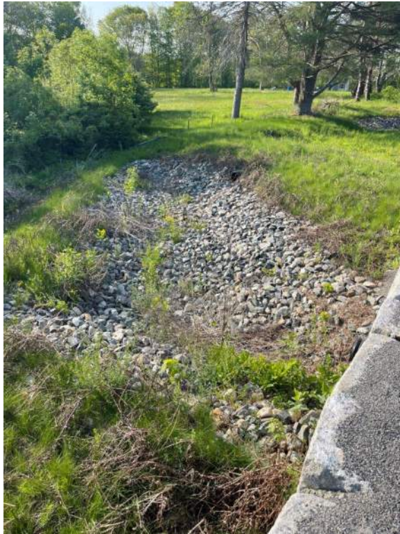
Pond 6P Outlet Swale
