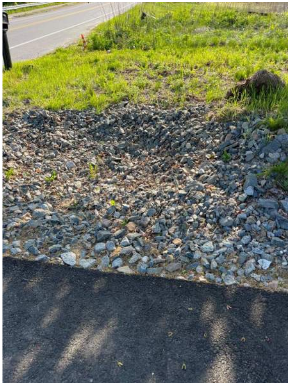
Common Drive – Plunge Pool – North Side
