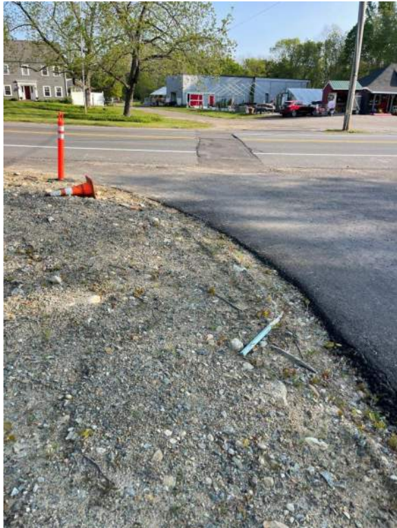
Waterline Connection in Main Street
