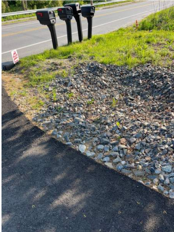
Common Drive – Plunge Pool – North Side
