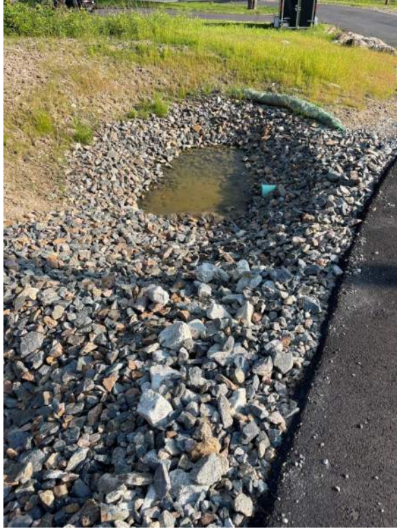
Lot 3 Driveway Rip Rap Swale Plunge Pool – South Side
