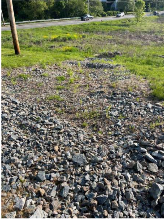
Common Drive – Rip Rap Diversion Swale #1 – North Side
