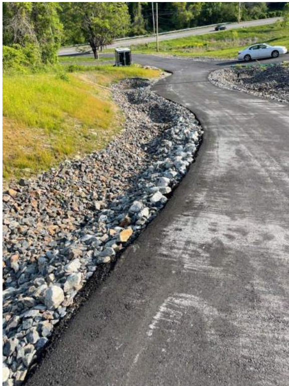
Lot 3 Driveway Rip Rap Swale – South Side
