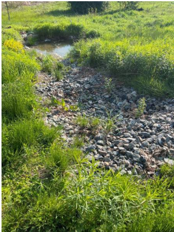
Common Drive – Rip Rap Diversion Swale #2 Plunge Pool – North Side
