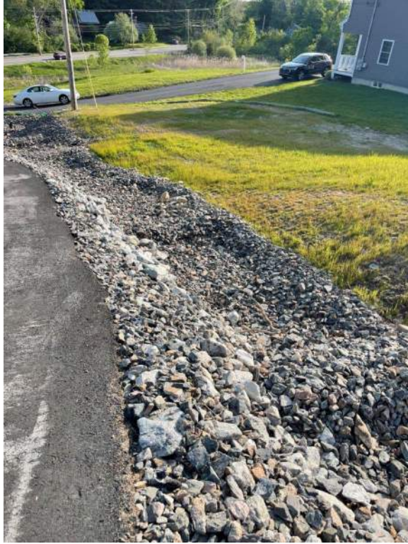
Lot 3 Driveway Rip Rap Swale – North Side
