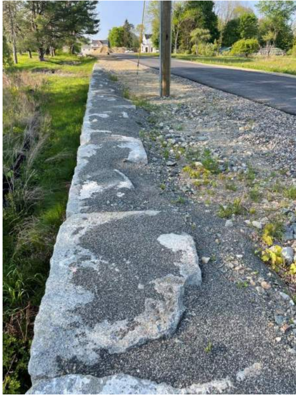
Paved Roadway, Retaining Wall and Pond 6P Outlet Swale
