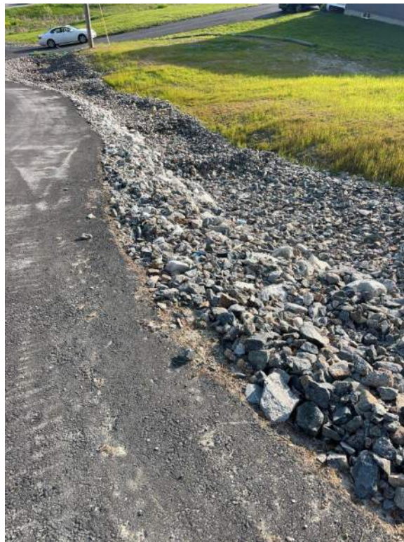
Lot 3 Driveway Rip Rap Swale – North Side
