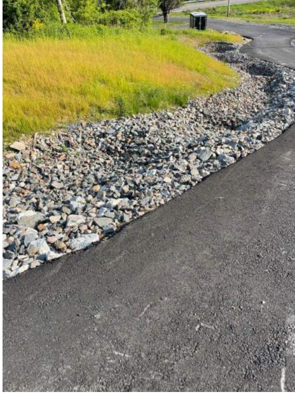
Lot 3 Driveway Rip Rap Swale – South Side
