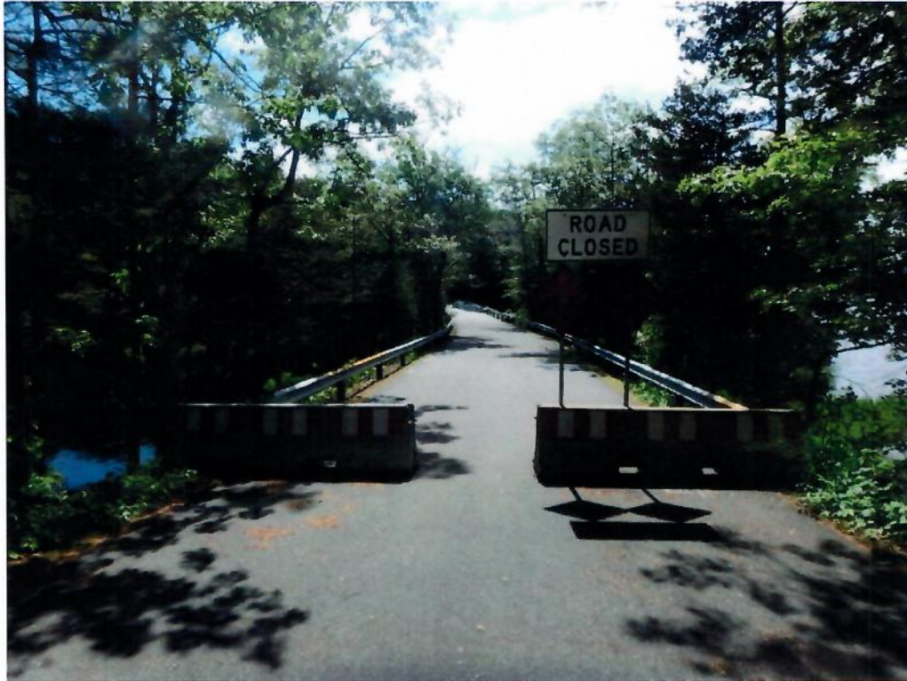
Photo 9: Road closed signs and jersey barriers installed at the west end of the bridge preventing vehicle traffic.
