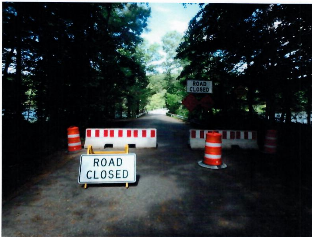
Photo 8: Road closed signs and jersey barriers installed at the east end of the bridge preventing vehicle traffic.
