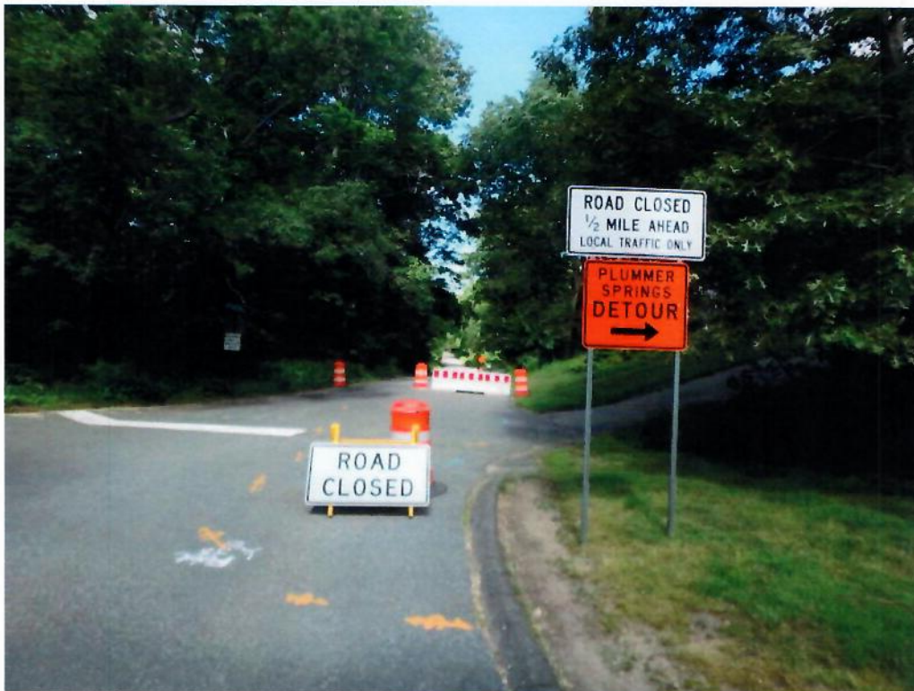
Photo 6: Road closed and detour signs at the intersection of Turkey Hill Road and Plummer Spring Road 1/2 mile east of the bridge.
