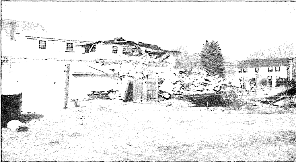
The Old building comes down –04/12/04
