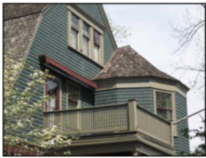
Example of windows, a balcony, and siding that would satisfy these Design Standards.
