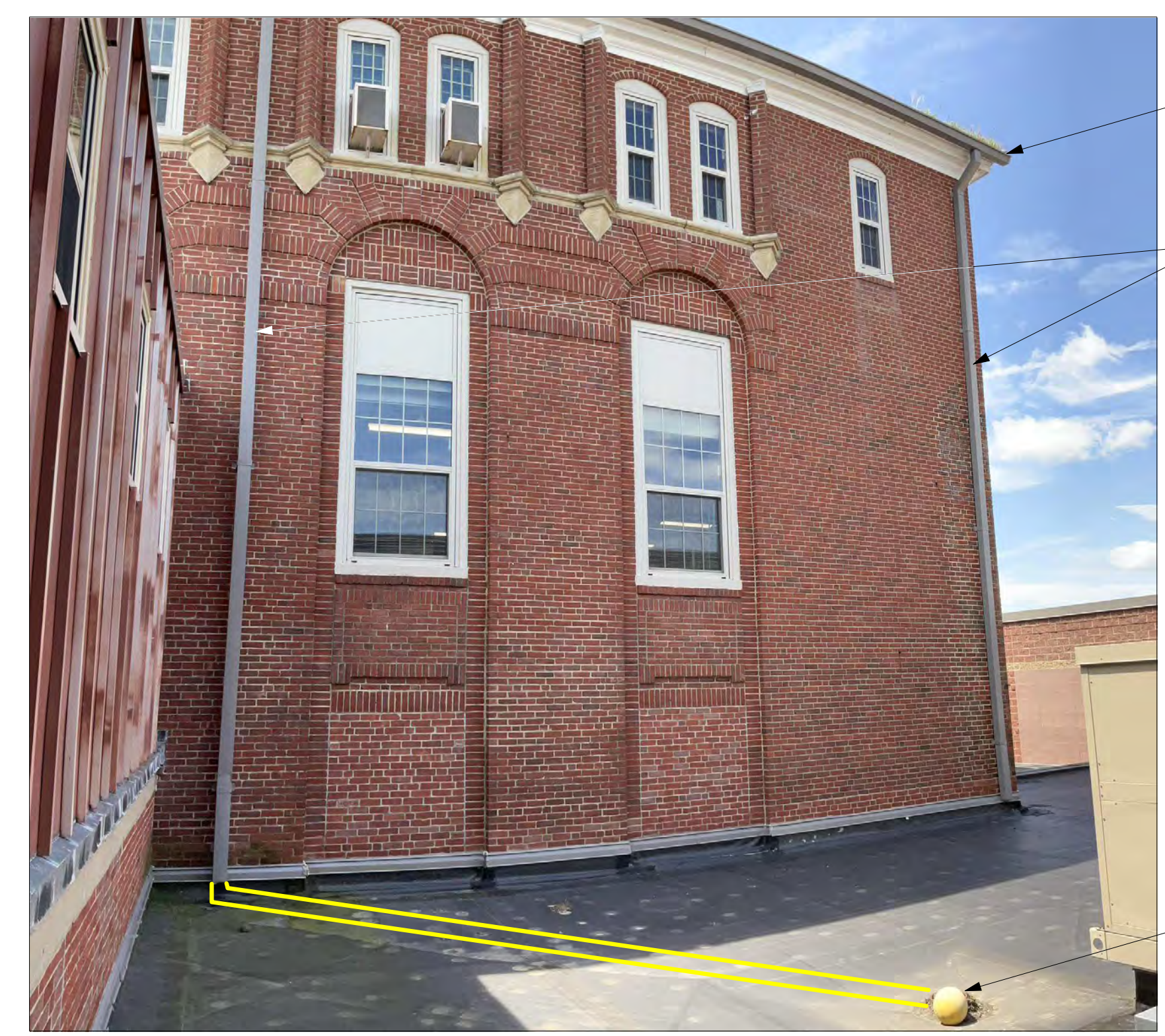
2 East Roof Downspout 1
