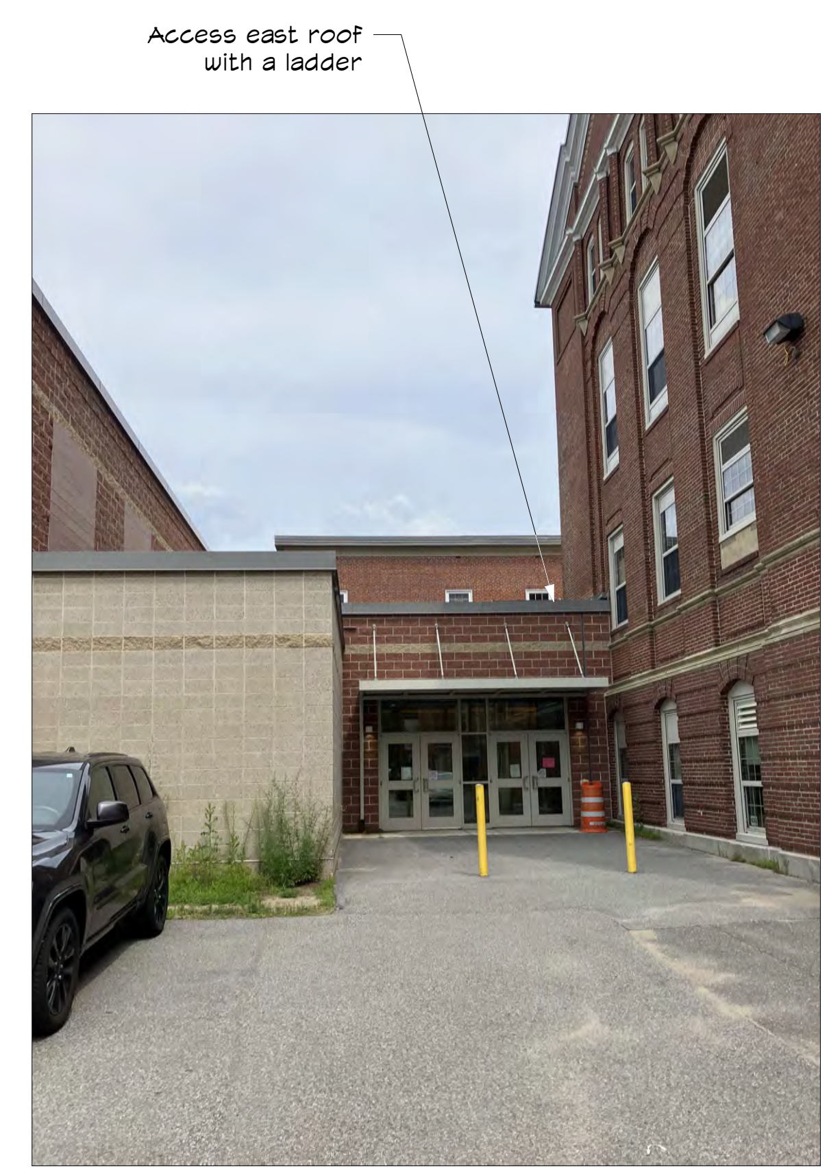
1 East Roof Downspout Location
