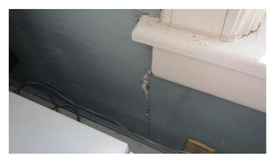
Likely water damaged plaster beneath window, likely from rain penetrating through/around window frame
