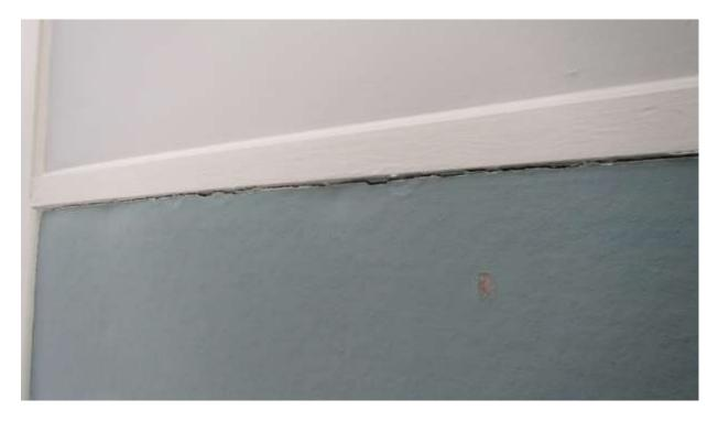
Crack between bulletin board frame and materials, possible odor pathway
