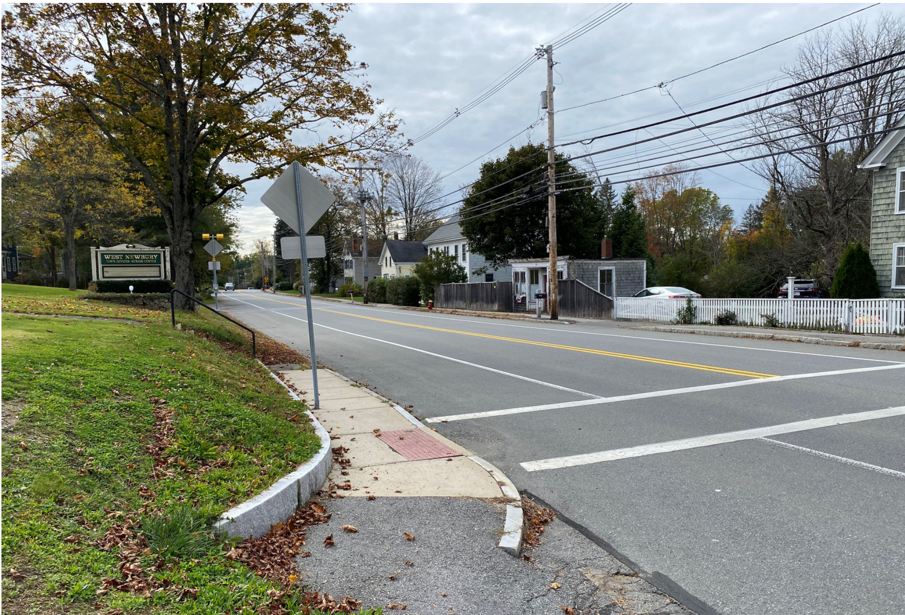
Image above: The crosswalks and signage around Town Offices were enhanced during Spring 2023. As part of the broader corridor study, this location and others will be considered for potential Rapid Flasher Beacons (RFBs).
