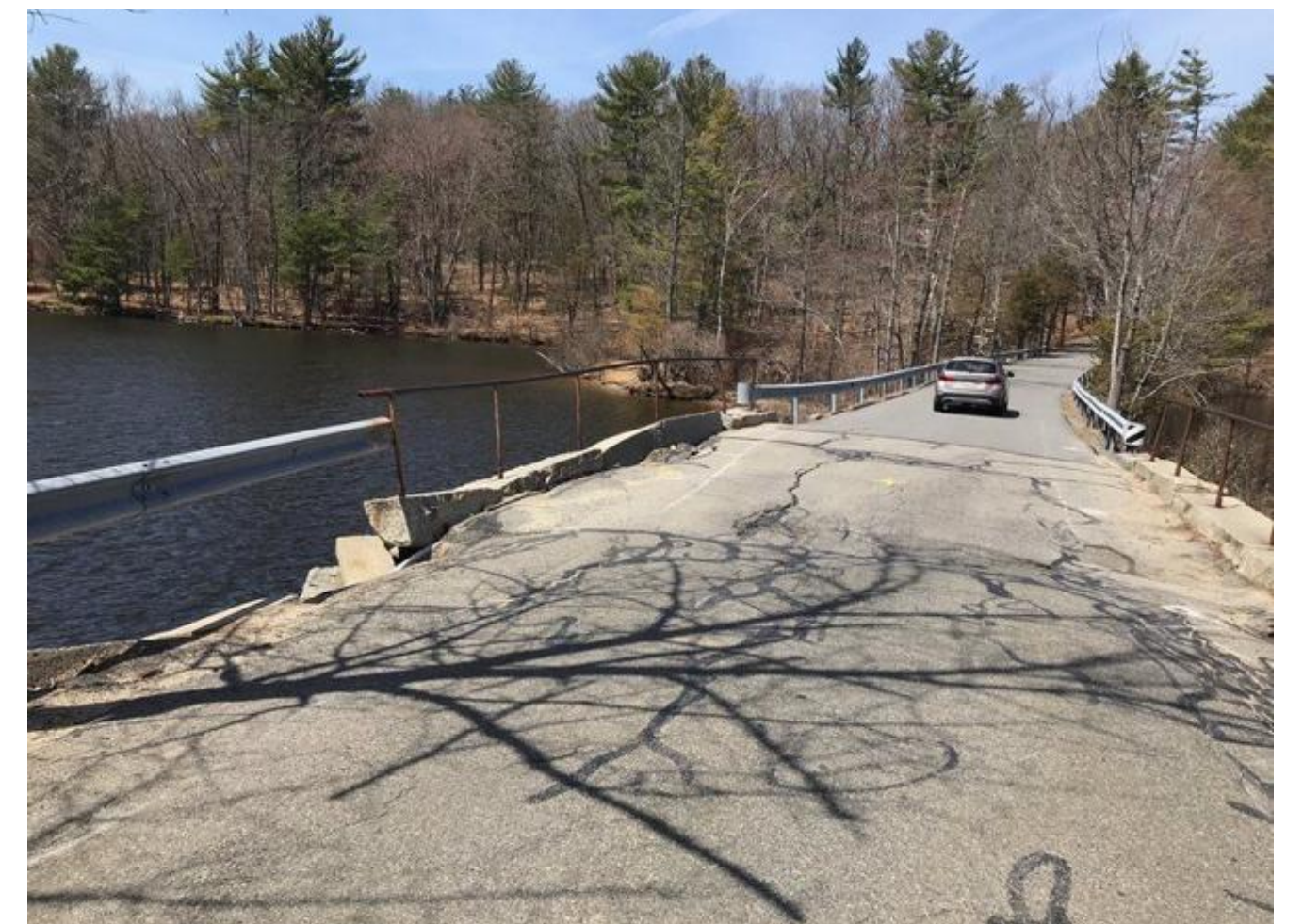
Above: An SUV traversing the Bridge prior to closure.
