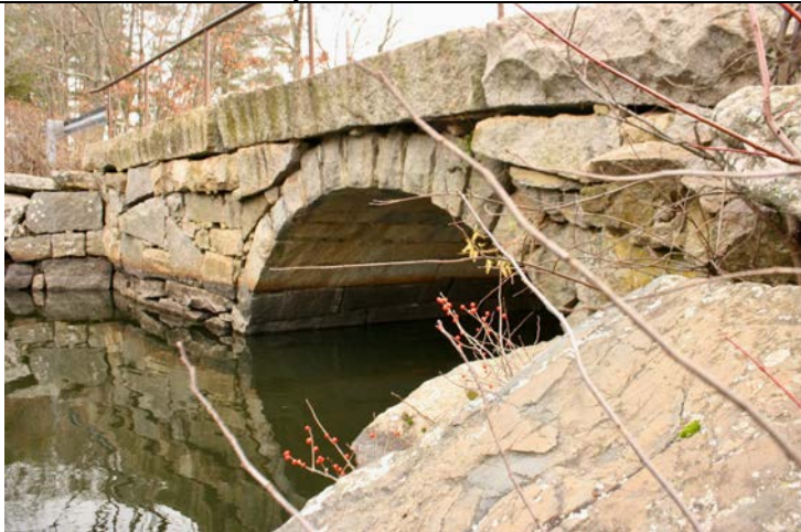
Photo 6. Detail of stone arch on north face of bridge, showing arch sheeting inside bridge.
