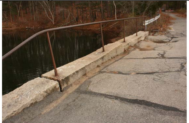
Photo 7. View of top of north side of bridge, showing cut granite blocks and metal pipe railing,
