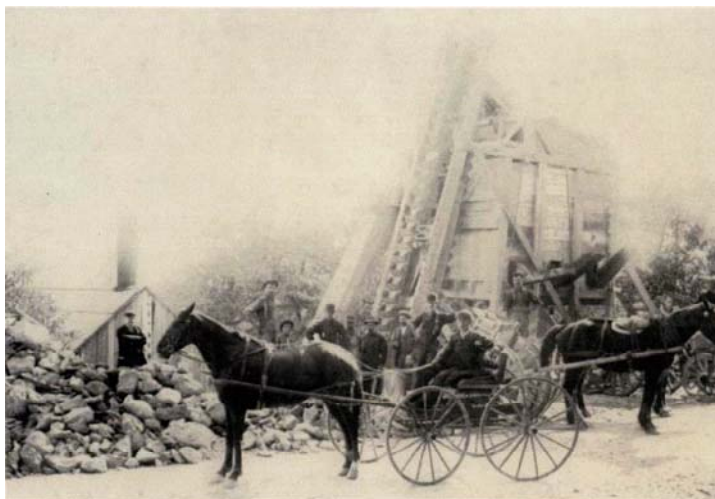
The crusher plant was on Pipestave Hill from Sept. 1896 to Oct. 1897 to crush rock for fill on Main Street. The road was being lowered to make it easier for electric cars to go up the hill on the way to Newburyport.
