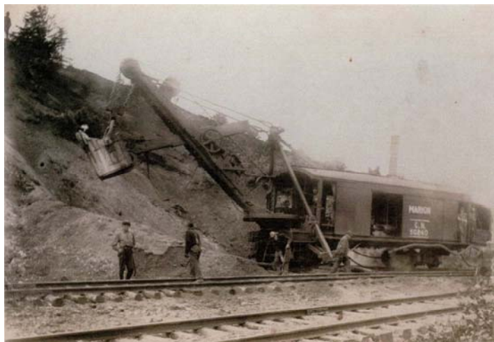
1896 – Pipestave Hill was cut down to ease the steep grade on Main Street. We have heard that farm workers on the estate would sit in the door of the stable with their legs hanging over the steep grade watching the road work. The stable was probably to the west of the Farmhouse (now a 4-unit apartment building) and is no longer there.
