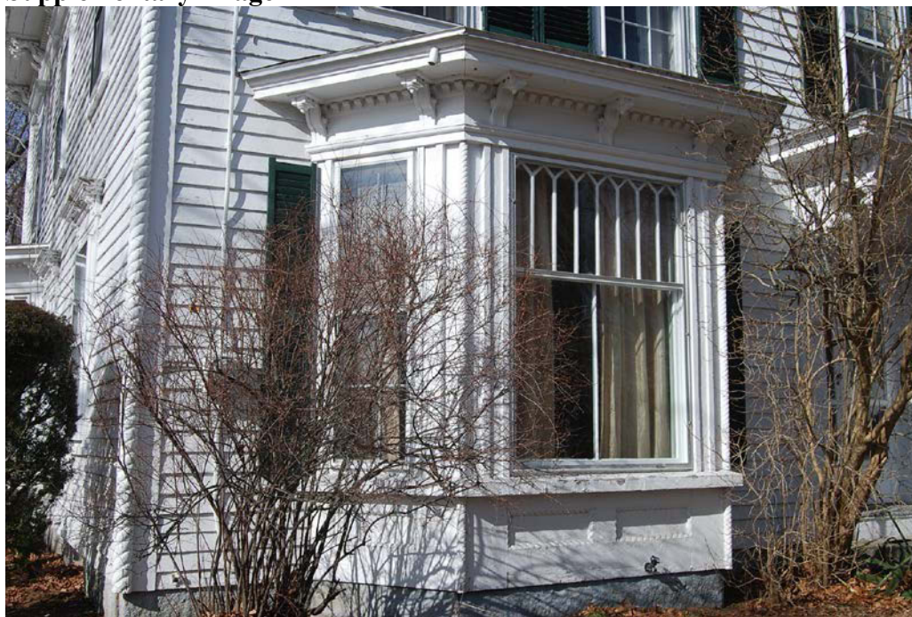
Photo 2. Bay window on façade. Note rope trim applied to cornerboards, used as mullions, and enclosing the panels on the bay window. Also note compound brackets with pendants and projecting hoods.
